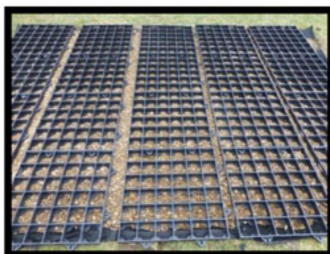
Lay the base in rows with small gaps
